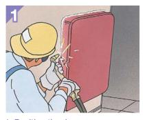
**1. Position the door.** Place the door frame at the appropriate site and tack weld it into position. Then solidly weld the frame to the surface.
