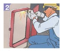
2. Cut the inside hole. Open the door and carefully torch burn the center to create the access area.
