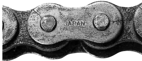
Hydrogen embrittlement cracking
